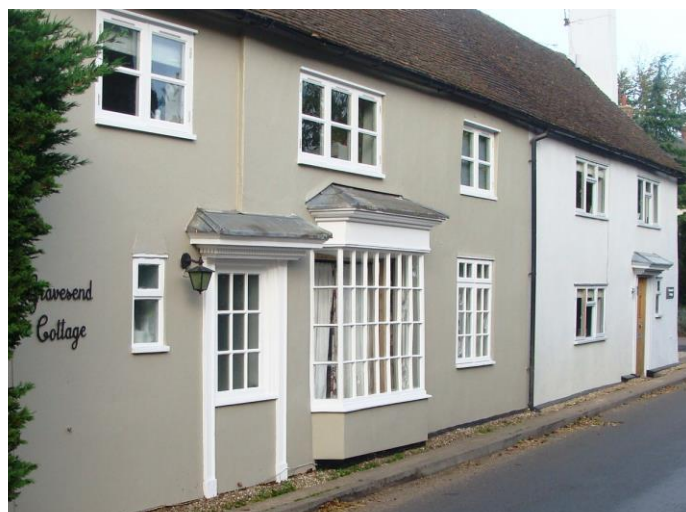
Picture 10: Gravesend Cottage and No.2 Gravesend Cottages make a significant visual contribution in the extended conservation area
