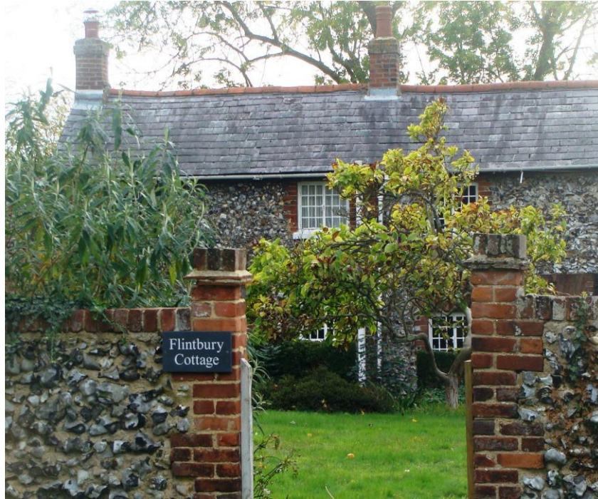
Picture 6: Flintbury Cottage, a charming 19 th century cottage of flint wall and slate roof construction. Boundary wall also included in listing
