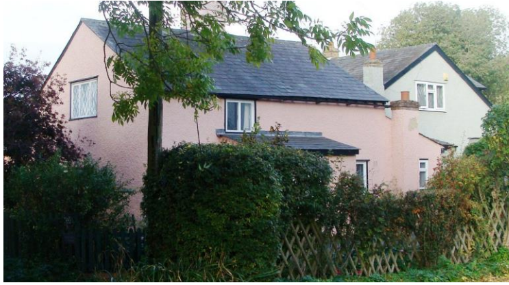
Picture 12: Hillside Cottage and Ashvale Cottage – Despite modern window and later additions this group is considered to be of sufficient architectural and historic quality to be retained and if possible, enhanced
